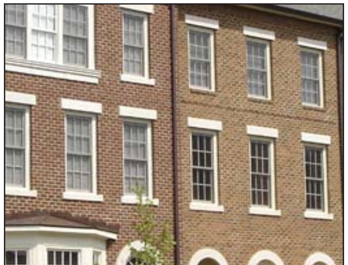
Example of gutter and downspout
