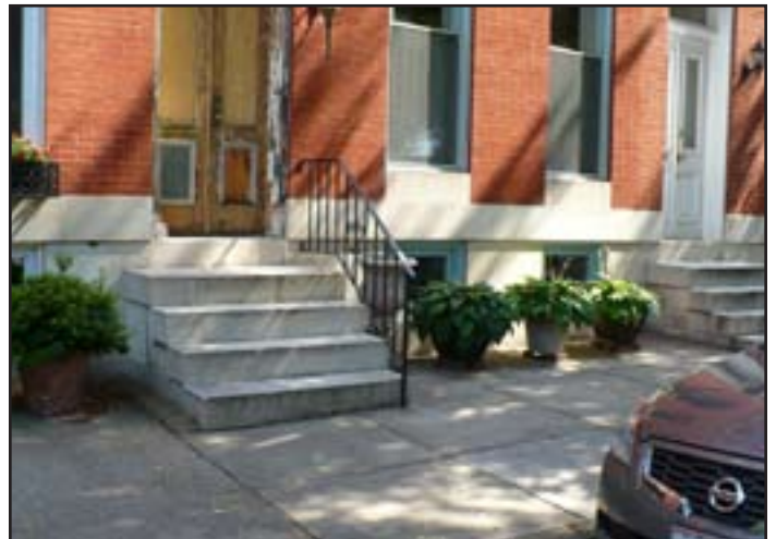
Example of precast foundation
