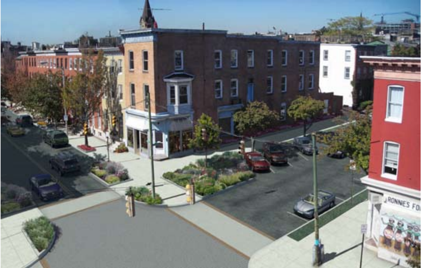
Phase 4: Stormwater runoff collection tree pits, continuous planting strips, and foundation plantings
