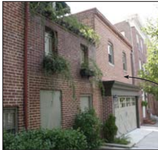
Addition compatible with existing structure
